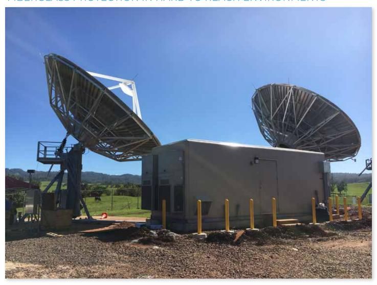
STS Global, a leader in satellite and terrestrial telecommunications systems, partnered with Shelter Works to deliver a rugged, insulated fiberglass equipment shelter for a Fixed Earth Station. The station, located high on a hill in Hawaii, supports two 9-meter satellite dishes servicing the island's television, Internet, and communications infrastructure.
