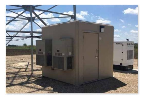
reaching 350 feet in height, required durable, weather-resistant equipment enclosures at their base to house sensitive digital radio equipment and the associated backup power systems.
