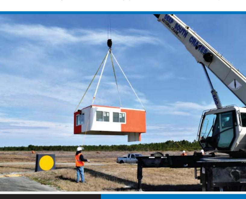
**Hurricane Resistant:** This particular coastal location is prone to hurricanes every year, so there was a requirement that whatever structure was developed needed to be able to withstand wind speeds of up to 140 mph (ours can withstand wind loads of up to 162 miles an hour.)
