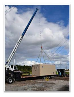
Shelter Works recommends that buildings be offloaded using an overhead crane or similar lifting equipment with sufficient capacity for the load.
