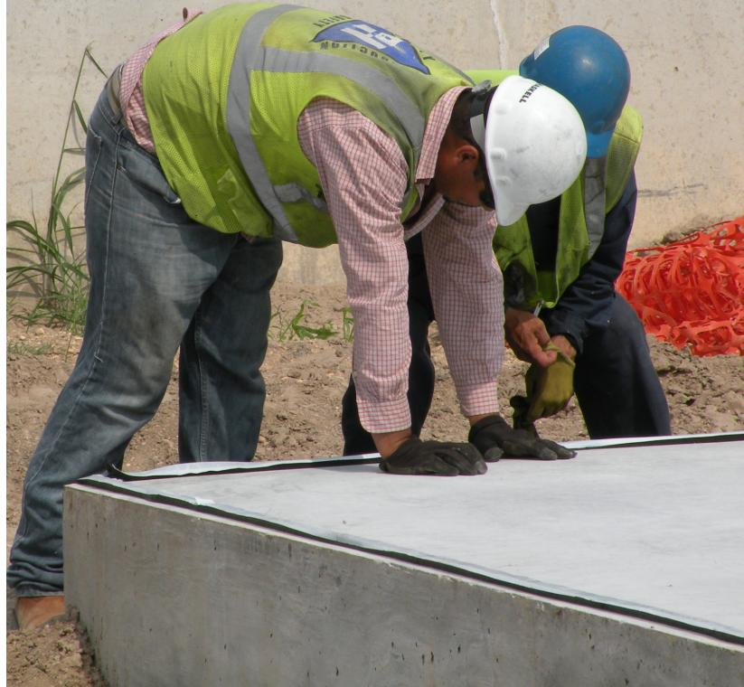
**(9)** Place alignment pins through the base flange and into the drilled holes in the slab at the four corners and at the midway point of each wall to guide the building down the remaining couple of inches onto the slab.
